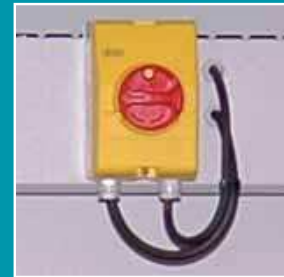
External local isolator
