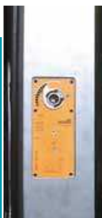
Actuator fitted and wired
